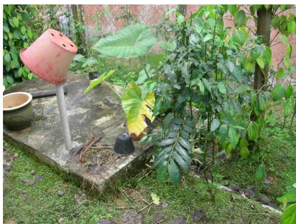
Figure 6.14 Septic tank (the pot is put on top of the aeration pipe to diminish the smell)
