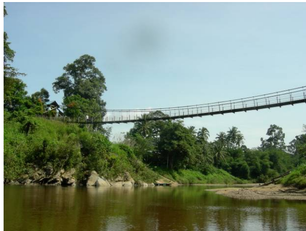
Figure 6.2: The extension bridge before entering the village on the left hand side
