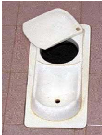
Figure 2.6: Squatting toilet with urine separation
